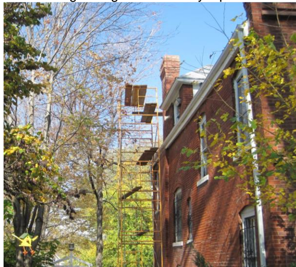
Scaffolding during west chimney top restoration
